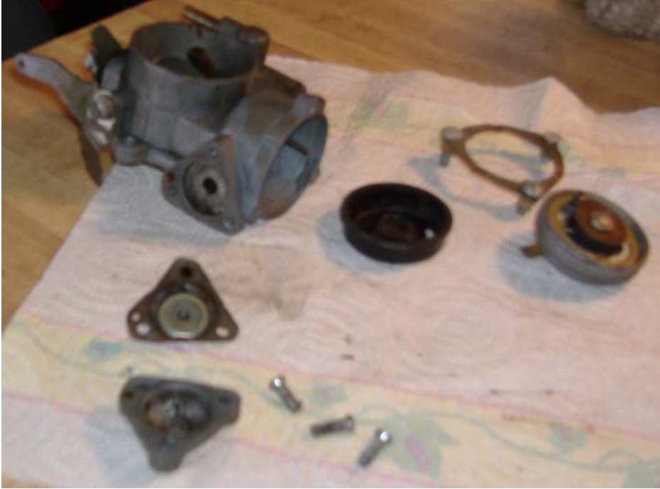
Figure 4 – Top Cover Parts Were Not Immersed; the Vacuum Diaphragm Was Worn Due to Age, not Exposure.
